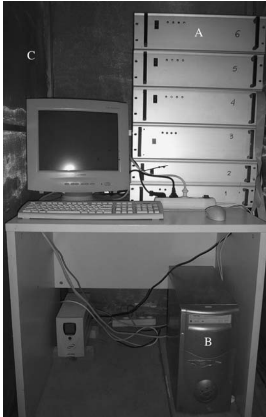
FIGURE 1. The Multi Channel Dynamic Exciter 100 V1 (MCDE). (A) Dipole antenna; (B) Pc's sophisticated program; (C) Faraday cage.
